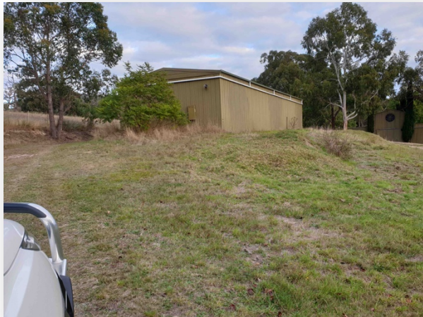
9 View southeast on accessway to sheds
