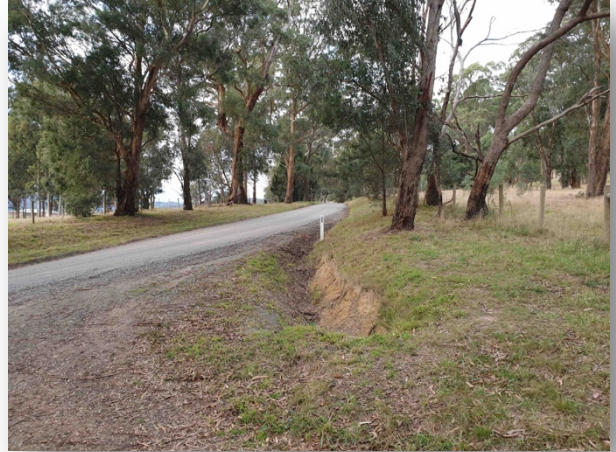
2 View northeast on Pinnacle Lane site entry on right
